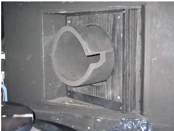
Figures 3 & 4: temporary insulation on the inside of the 2dcoude collimator mirror housing
